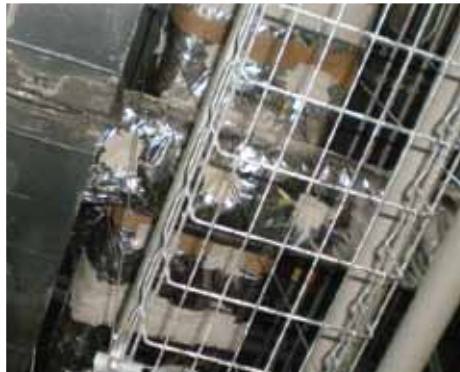
Trapeze hangers with strut
