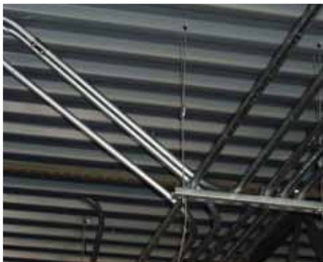
Trapeze hangers with strut
