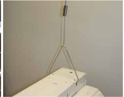
Standard Gripple HF with V-Brackets
