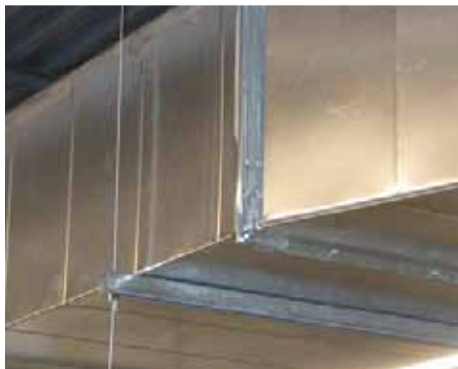
Trapeze hanger with struts
