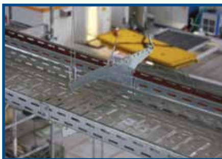
Cable tray with G-Bracket
