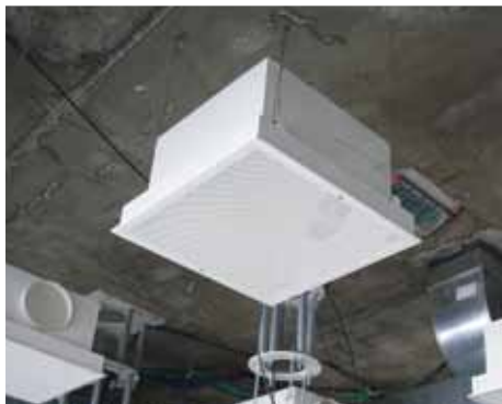
Hangers attached to brackets
