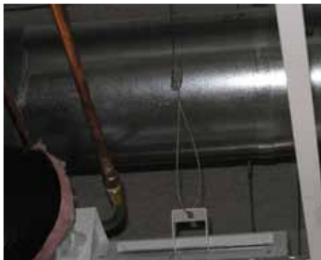
Hangers attached to brackets
