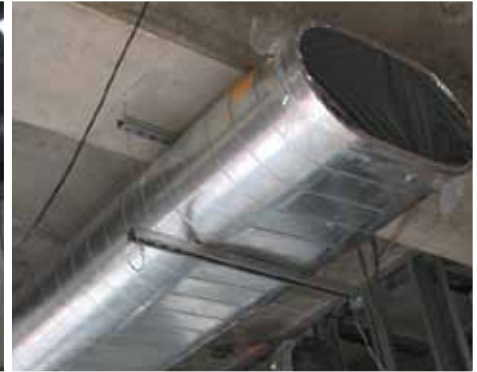
Trapeze hanger with strut
