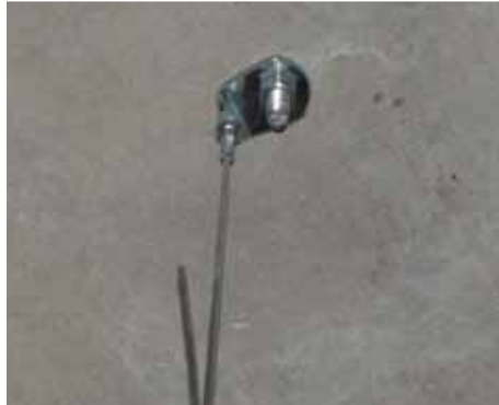
90° Eyelet in concrete
