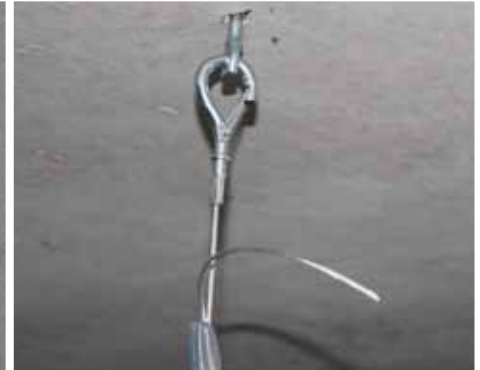
Hook in concrete ceiling anchor
