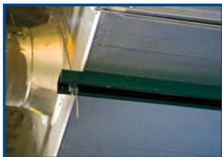
Rectangular duct with strut
