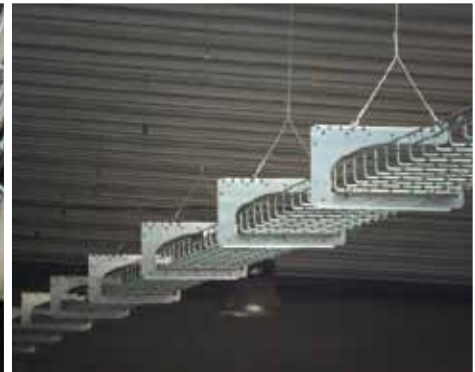
Y-Fit hanger with G-Bracket
