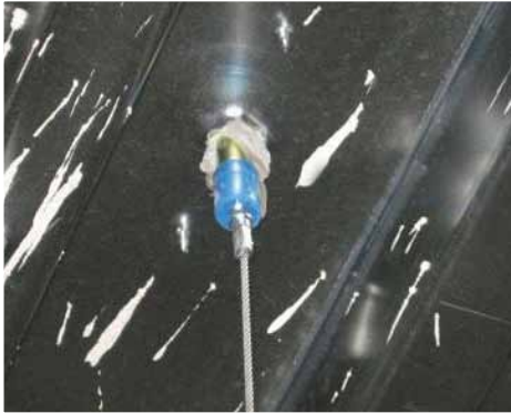
Stud in concrete insert
