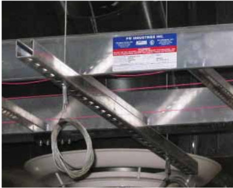
Trapeze hangers with strut
