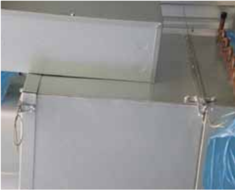
Duct trapeze hangers
